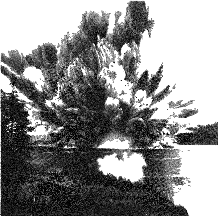
Fig. 2.9 Ripple Rock, in the Seymour Narrows, British Columbia, is destroyed by a single charge of 1400 tons of chemical high explosive.
